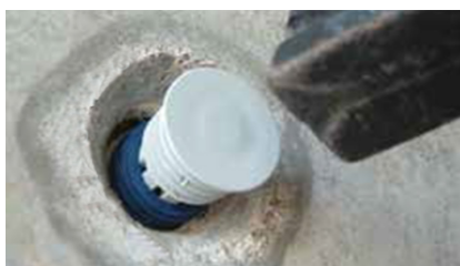
Hammer the Sealing Plug into the formwork spacer
